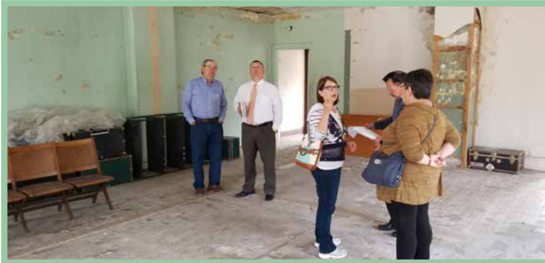
MTHS board members visiting the upper floor of the old firehouse. Shown are. L-R. Paul Schreiber, Ron Knaus, Fay Walker, Jim Schaefer and Rachel Muchin-Young. Others present included Andy LaFond, the director of public works for the village, historic contractor David Salvaggio, village trustee Rob Holyoke, TBA executive director Rob Kos, and MTHS board members Doug Hansen and Bob Blazich.
